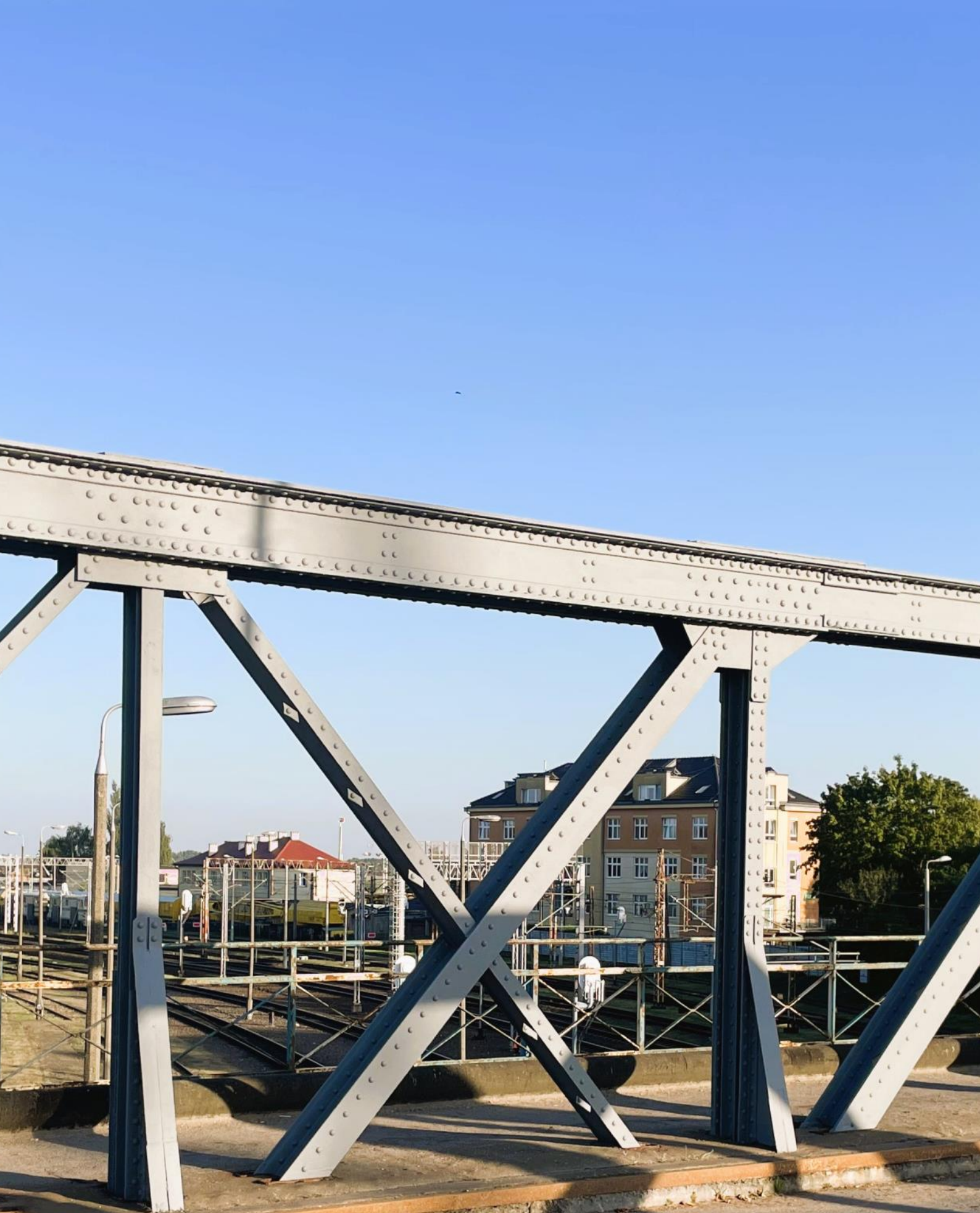
Restoration of a 120-year-old historic bridge with CREBONIT Hybrid System
